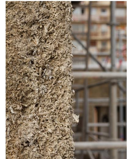
Fig. 15, 16, 17 and 18 - Hempcrete is a compound, an assembly of hemp shives (the aggregate) and lime (the binder) which is only formed at the moment of its implementation by the operator. It does not exist prior to its instantiation on the construction site. The projection of the hempcrete into the wall, by agglomeration, reveals the conditions of the final continuity of this mass.
