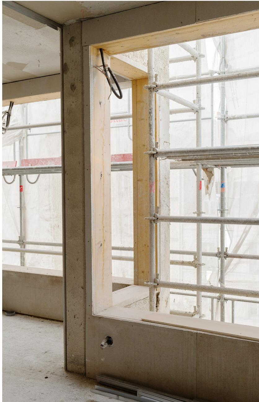
Fig. 2 - The hempcrete is the whole envelop of the building. The insulation is the whole wall.
