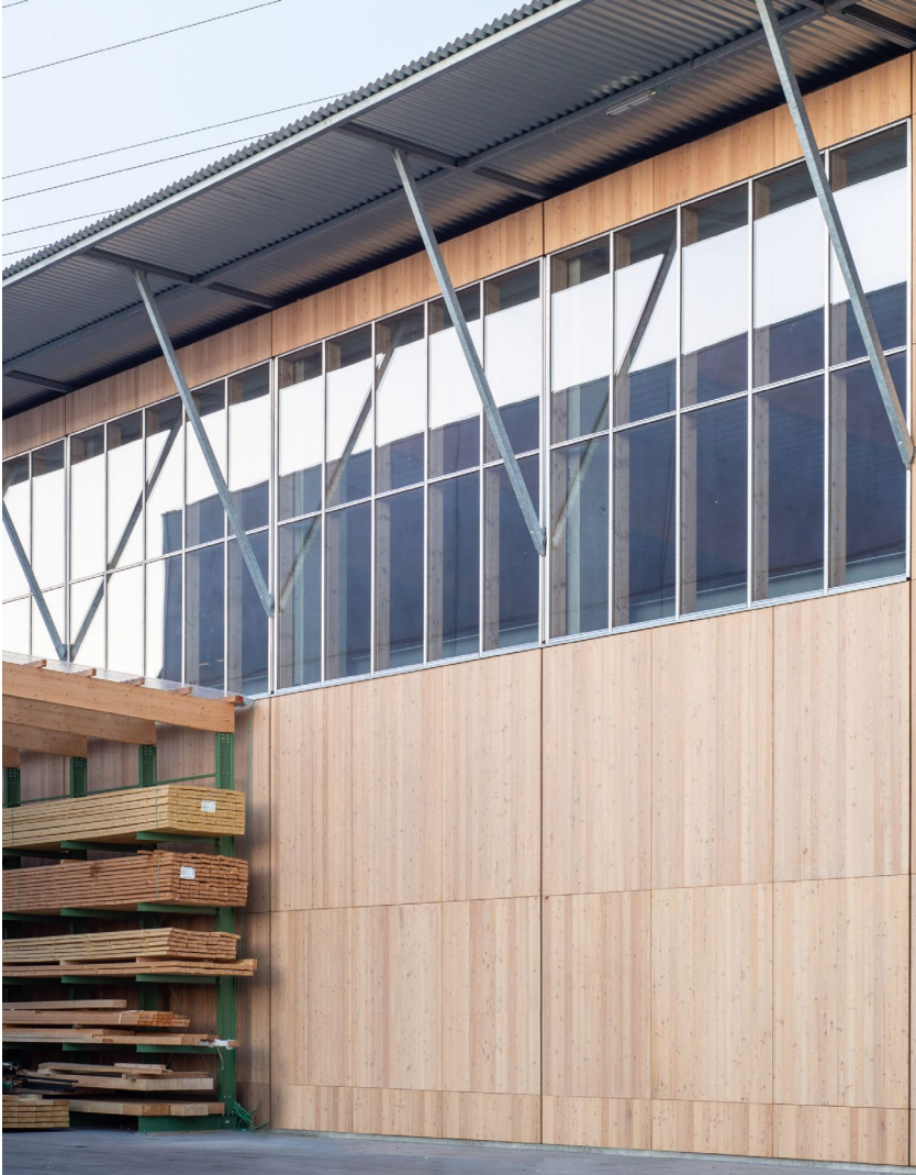
G1812, Industrial building (Construction), Ghent (2018-...), GAFPA
