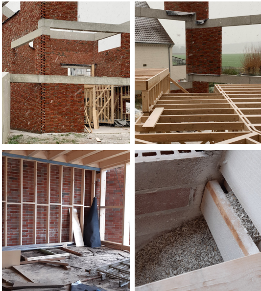
The construction of the jtB house Brick shell and timber frame, limehemp insulation with no ventilated cavity (right)
