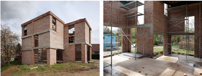
'The Future Ruin' (l'abri souverain) of dnA house, exterior (left) and interior (right) Photos Stijn Bollaert
