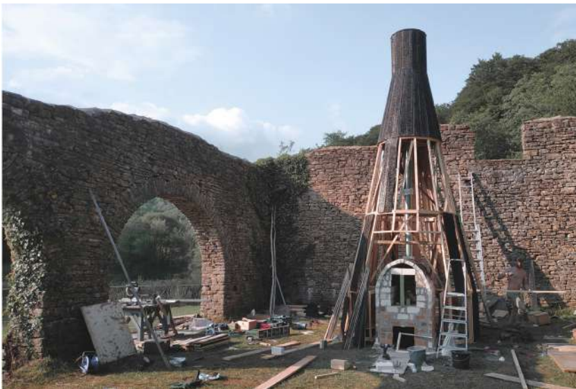
Fig.14 - The hoven being built
