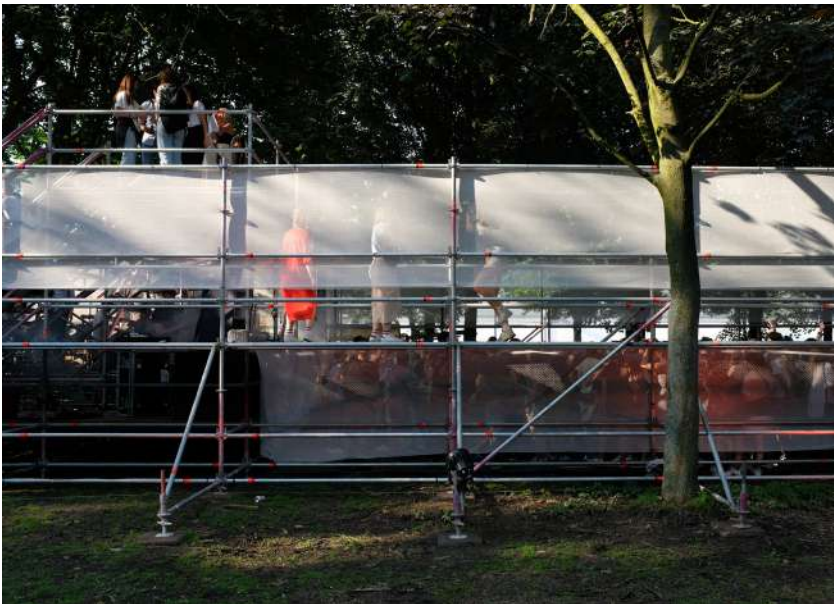
Contraic Open Air, June 2019
