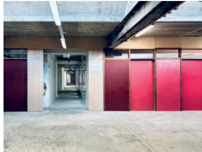
A series of reused doors composed into an interior division wall.
