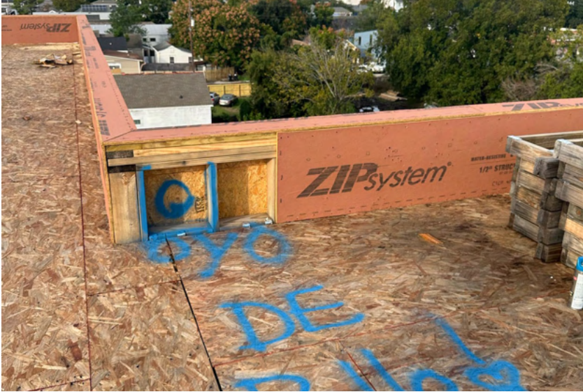
Fig. 1 Scupper rough opening on roof with blue spray paint marking the opening and the words “oyo de pollo” listed below ending with a heart shaped exclamation mark. The mark is half joke and half technical “oyo” is misspelled but should be “hoyo” translating to hole.
