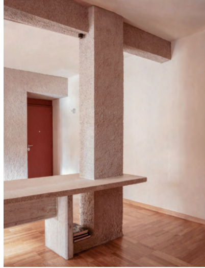
Fig. 4 Quattro spazi | The final result of the close collaboration between the carpenter, the flooring installer, the painter, and the architect, where traditional plaster techniques are reinterpreted to create an accent that emphasizes the structural presence of the column wrapping around the table.
