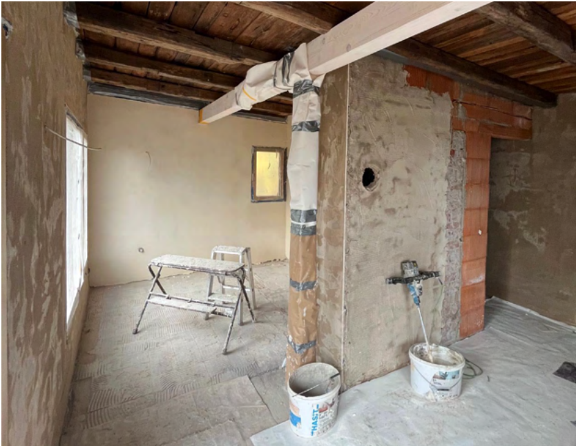
fig 8.: the adapted column, carrying the weight and wrapped for protection.
