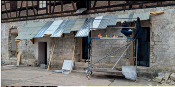
8th of July 2025 - Construction of the roof with discarded garage gates
