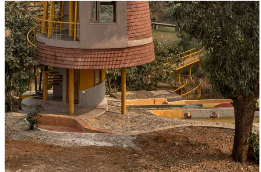
4th May 2024 . Inside the master bedroom's seating section, at the corner between the bedside table and the rotating door, there are two skylights - one in the roof and another in the floor. Each casts light onto the other, eventually illuminating the sloping contour. It brings to mind the moment when light first touched the ground before the building was constructed.
