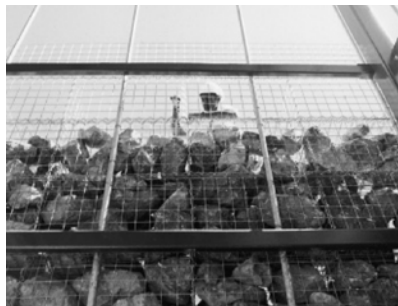
Construction process filling up the gabion walls Herzog and the Meuron's project Dominus Winery .
