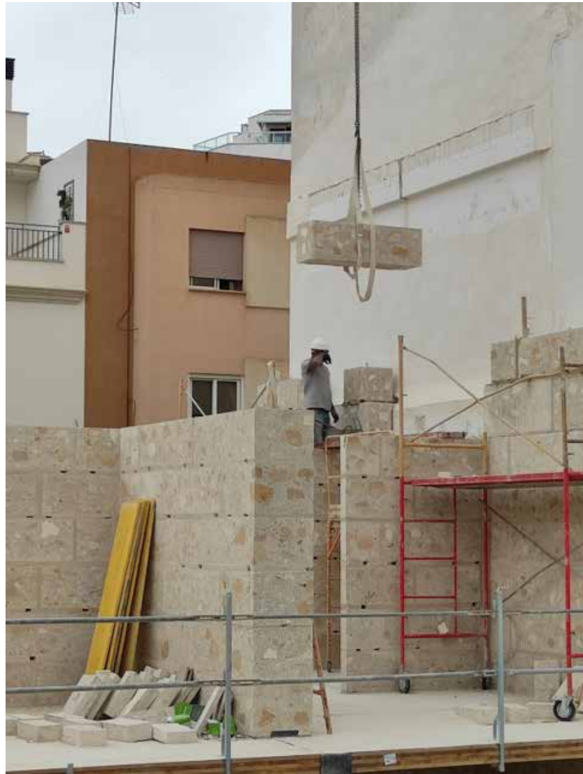
Construction site. Photo by Harquitectes
