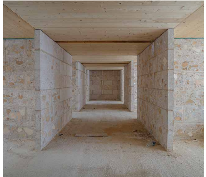
Social housing 2104, the final structure. Photo by Harquitectes
