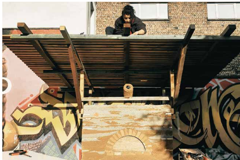
Maria Glionna building a pizza oven made of earth and reusing materials.
