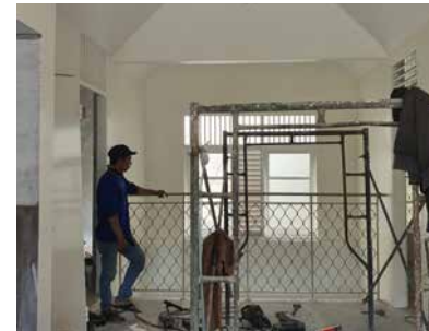
Figure.3 Repurposing building element to be used as another function : window bars remodified and transformed to be railing for the new void. Reused the old existing windows and doors by repainting and placing to the new arrangement of rooms.
