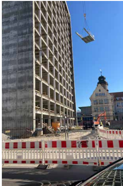
Replacing the old façade
