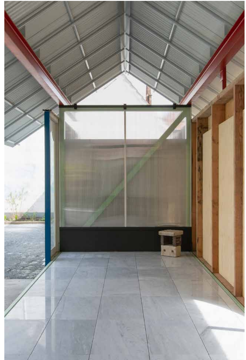
Fig. 7. Norell/Rodhe, Raamland (2024). The pavilion included wall panels from an abandoned club in Oostende, second-hand Carrara tiles from Brussels, wood used at previous triennials and inert materials from industrial recycling centres.
