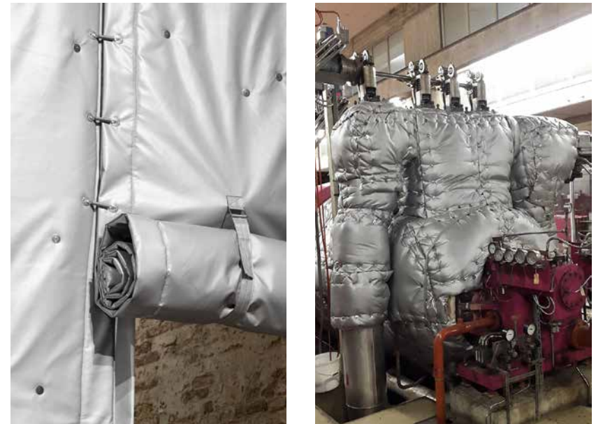
A Comparative Dialogue Act , 2024, Every Island and Andrea Mancini, Luxembourg Pavilion Venice Art Biennale: Top and bottom left: View and details of the insulating curtain main facade. Photography by Delfino Sisto Legnani. Bottom right: an example of an insulating jacket for industrial machinery.
