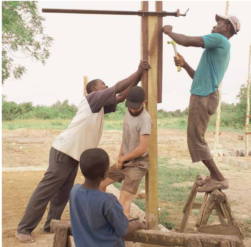
Corentin Dalon, architecte supporting the work of an artisan carpenter during the construction of the Children Center Xewa Sowé in Bénin.
