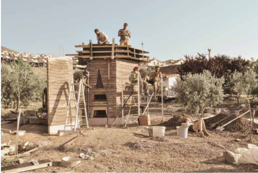
Participatory site led by Timur Ersen ( Atelier KARA), earth artisan who was once an architect.
