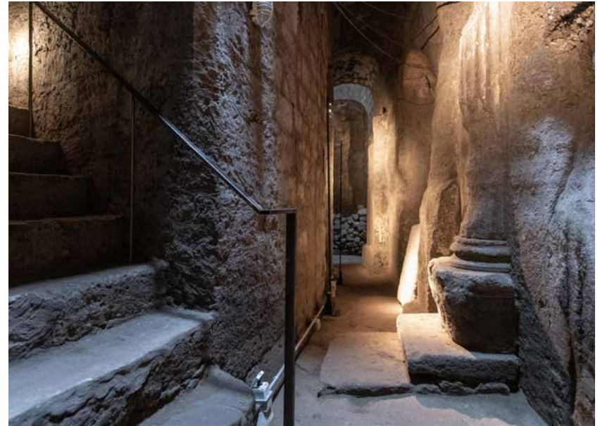
Fig. 5 Access staircase to the Greek necropolis, with black steel railing. The intervention facilitates visitor movement while preserving the raw quality of the excavation. Archaeology remains the protagonist, guiding the design approach.
